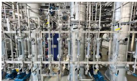
The five distillation columns for Swiss ethanol in the production hall of the sugar factory in Aarberg, Bern.
